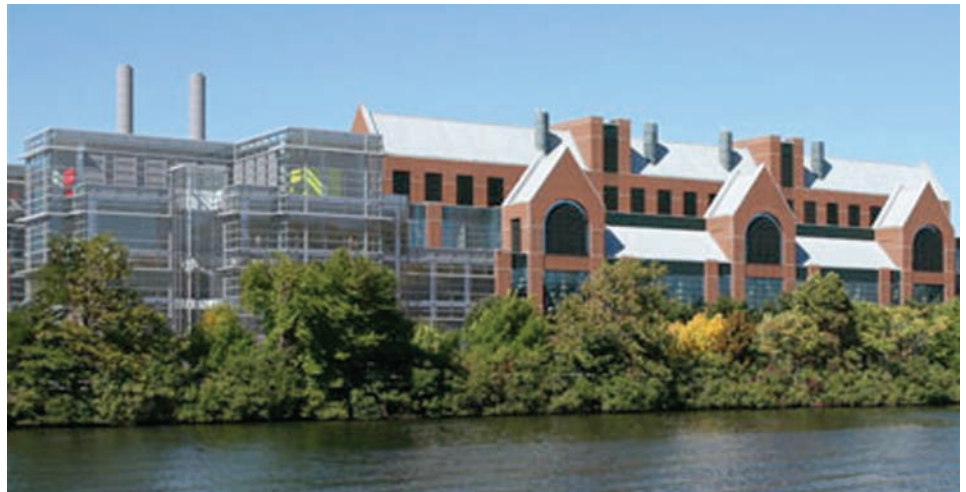
Genzyme Corp. manufacturing plant, Allston MA
