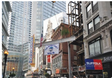
Modern Theatre topping off, Boston MA
