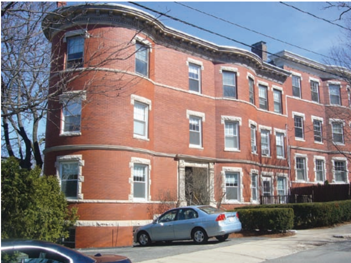
8 Colbourne Crescent, Brookline MA
