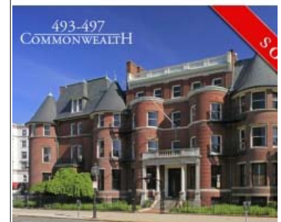
493 Commonwealth Ave., Boston
